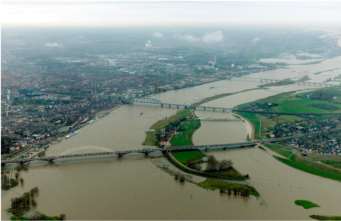
Figure 10. Bypass in the Waal river at Nijmegen (copyright RWS).
